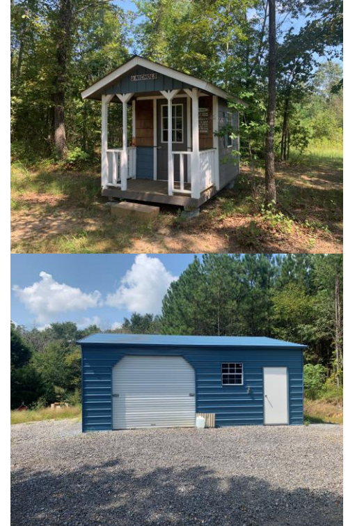
Existing Structures with Utilities
